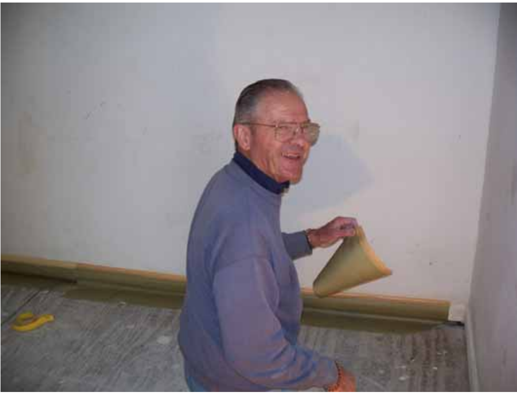
Veronica Stevenson's house: Baseboard prep before Ed Kalenda's texture coat.
