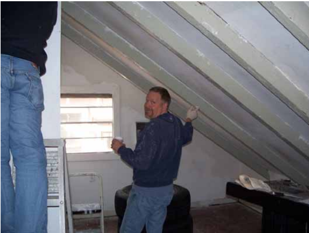
Veronica Stevenson's house: Wall and ceiling prep before texture coat.
